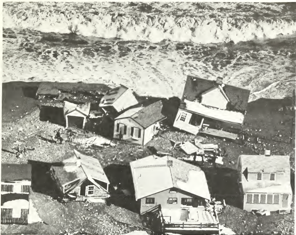
FIGURE 151B.—Section of shoreline at Scituate-Marshfield, Mass., showing the extensive tidal flooding damage to homes caused by the combination of strong onshore winds and the elevated perigean spring tides of February 6-7, 1978 associated with the pseudo-perigee-syzygy alignment of 1978 February 6, P-S = -42^{\circ} . (See item 10.)
